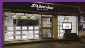
Double fronted office
